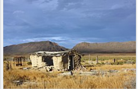
Derelict building off State Route 305 in the Reese River Valley with the Shoshone Range in the distance
